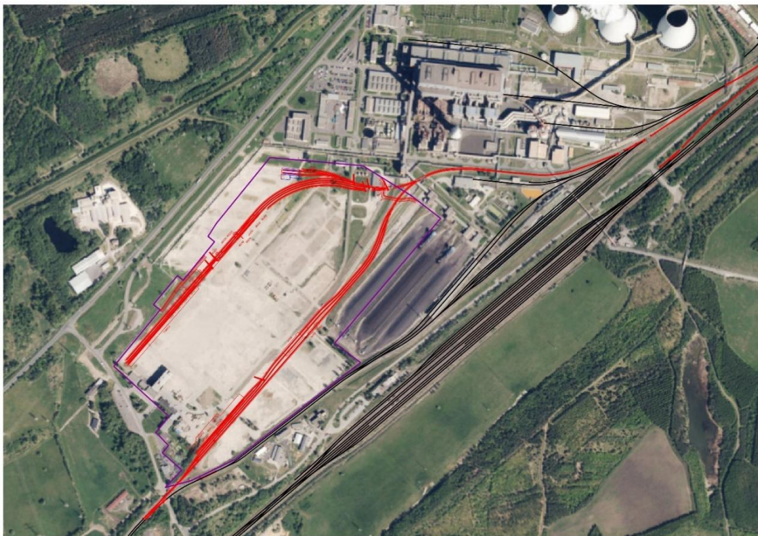
Figure 10: Railway siding at the Pruněřov processing plant
